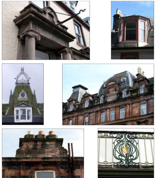
Figure 32: Top: Georgian refinement in the Ionic porch in Castle Street; (right) bay dormers are a strong feature of the Victorian era; Centre Victorian flamboyancy: French Pavilion Roofs: (left) Victoria Hotel; (right) the Duncan Halls; Below: Classic refinement displayed on a carved chimney head in High Street; (right) decorative Art Nouveau iron work on the Winter Gardens,
