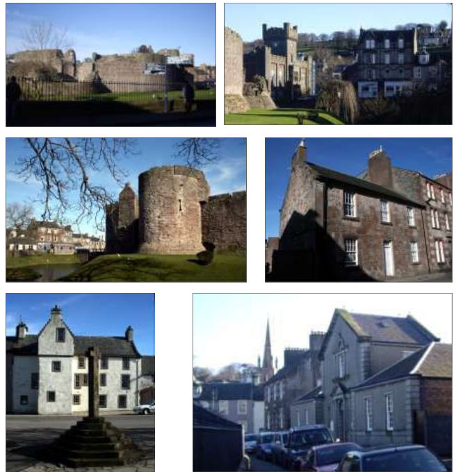
Figure 17: Top (left) the circular curtain wall of the castle; (right): view east to the former County Buildings and a tall tenement on the corner of High Street and Castle Street. Centre (left): the castle's remaining drum tower, low domestic buildings on Castlehill Street beyond; (right): No.4 King Street an early townhouse (1749); Below: (left) former Stuarts' Townhouse and market cross; (right) Bute Museum and No.3 Stuart Street.
