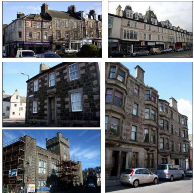
Figure 30: Top: mixed use flatted buildings are typical of the Character Area, such as the tenements on High Street with residential accommodation above and a mixture of retail uses at street level; (right) hotels follow this pattern, the Victoria Hotel has its entrance and shops at street level. Centre: (left) sole residential use for example a flatted house in Stuart Street and tenements in Bishop Street; Below: the former County Buildings being converted to residential use.
